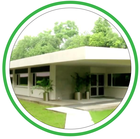
LC 3 Building Made in Swiss Embassy, India
